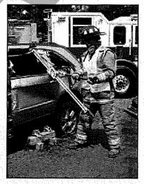
**Step 8:** Operate the jack to push the door down and off the latching mechanism.
