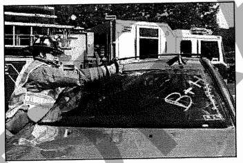
Step 3: Cut the glass at the roof line to connect the side cuts.
